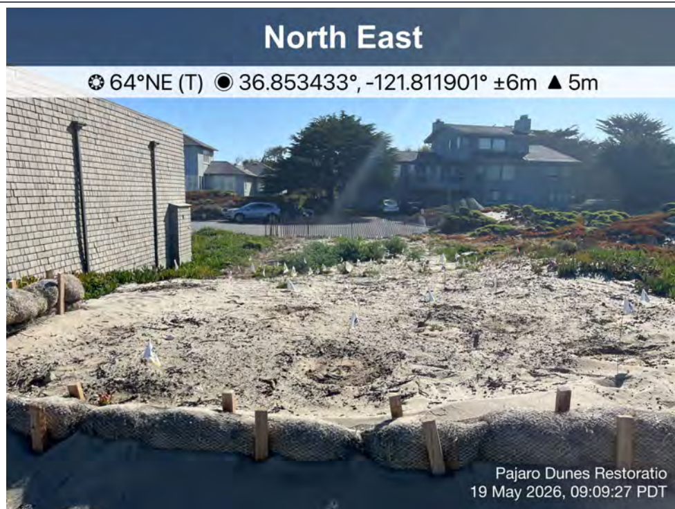
Photo 6. Viewing northeast at the straw wattle barrier surrounding the top western section of the project site at Photo Point 3.
