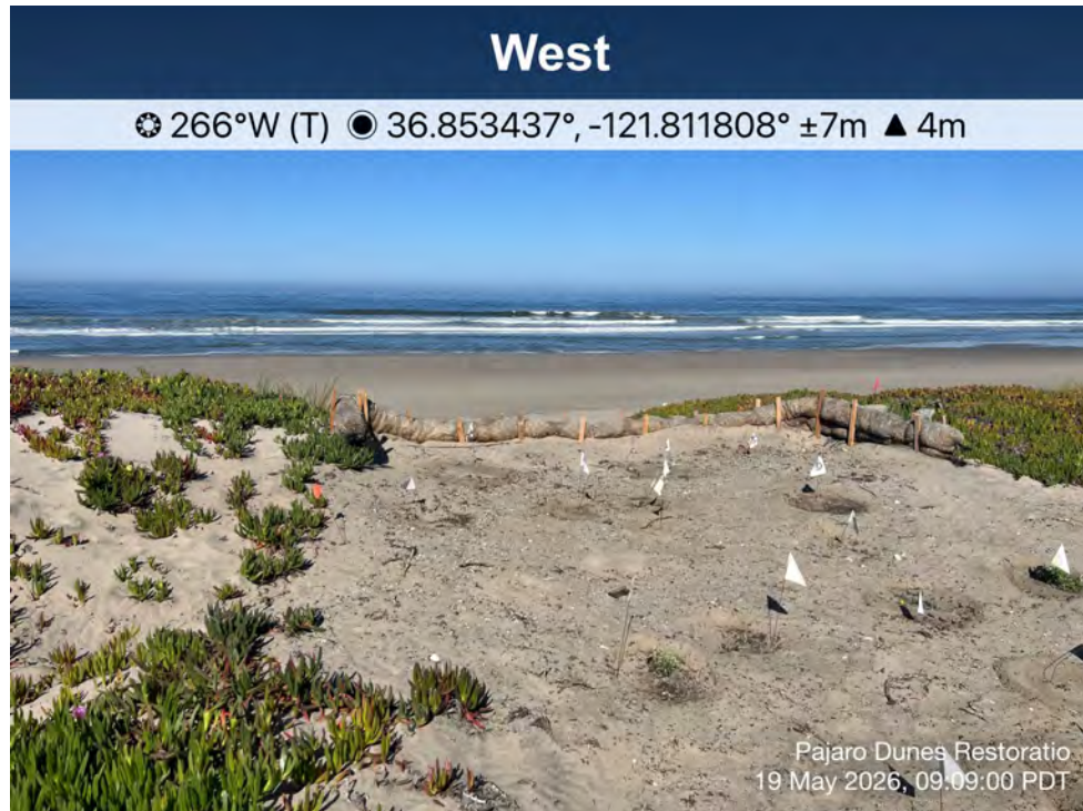
Photo 5. Viewing west at the straw wattle barrier surrounding the top western section of the project site.
